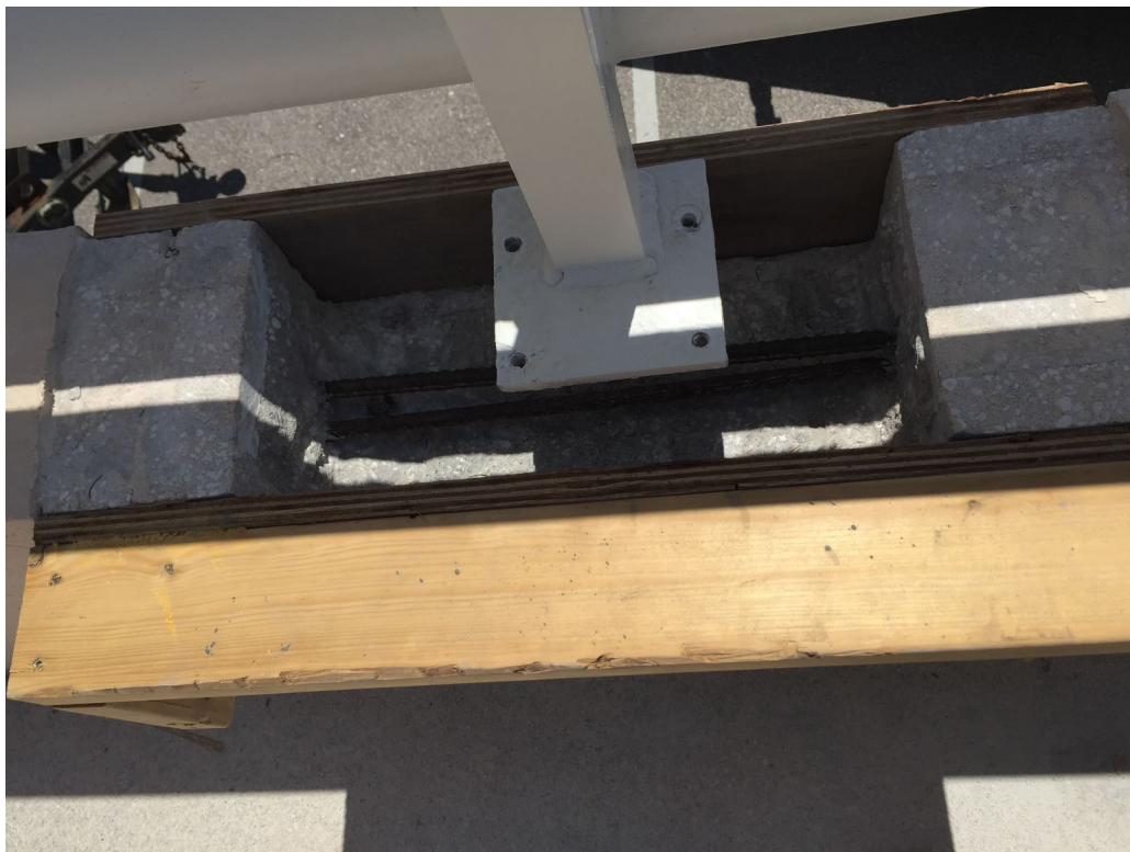
Picture 4: Completed excavation on knee wall
