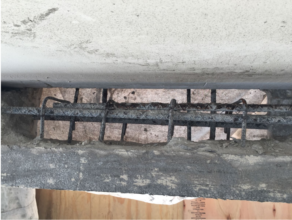
Picture 1: Completed excavation, sandblasting in-progress
