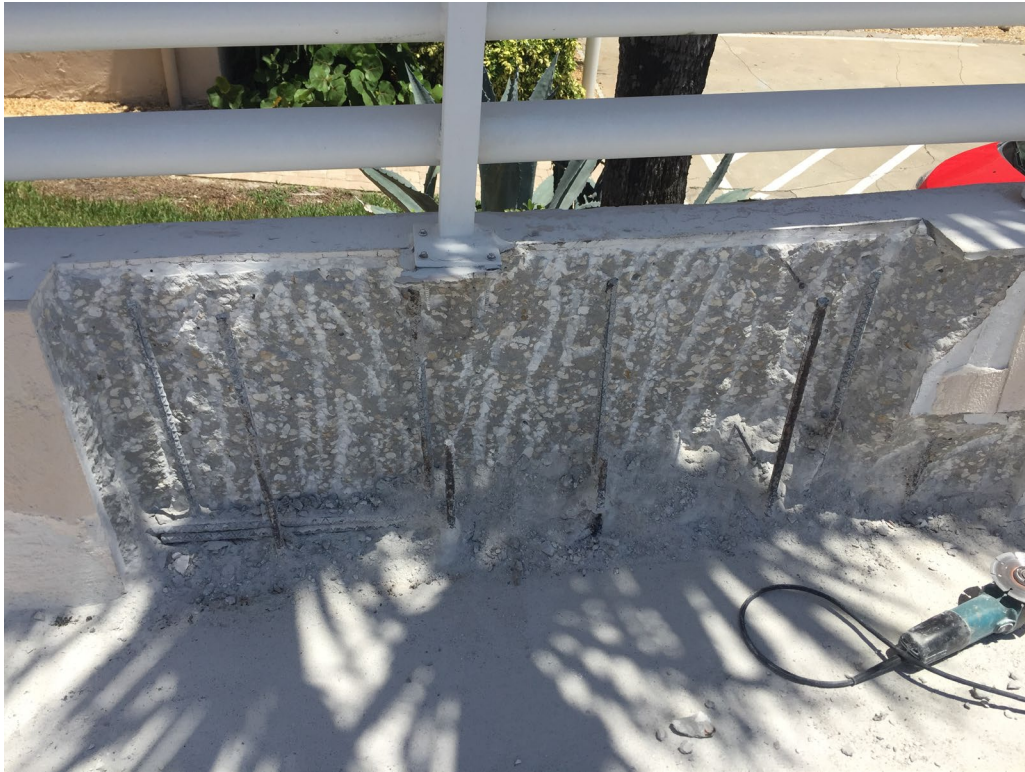
Picture 3: In-progress excavation on knee wall
