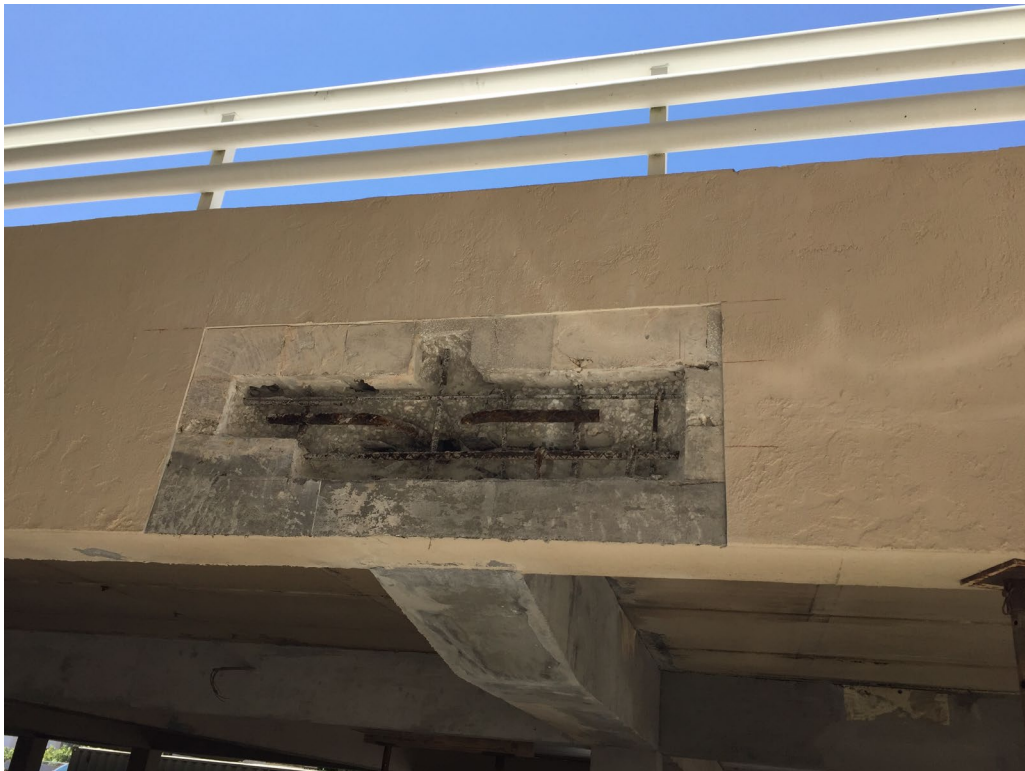
Picture 2: Completed excavation
